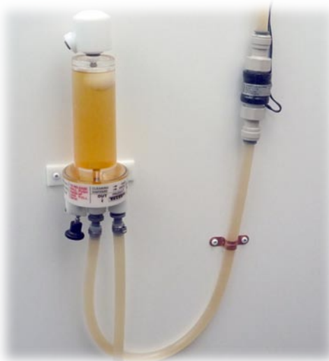
Figure 3 Flow meter with FOB
