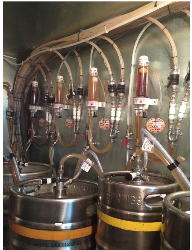
Figure 7: flow meters in teed beer lines
