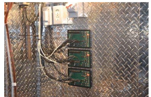
Figure 5: flow meter collector boxes without cover for 48 flow meters
