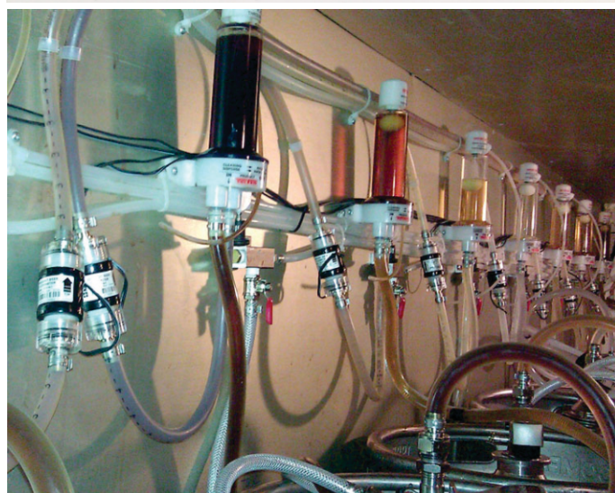
Flow meters and FOBs in beer cooler with cables.
